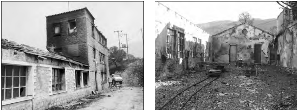
Figures 2a and b. External and inside view of the timber sawmill after the fire.
