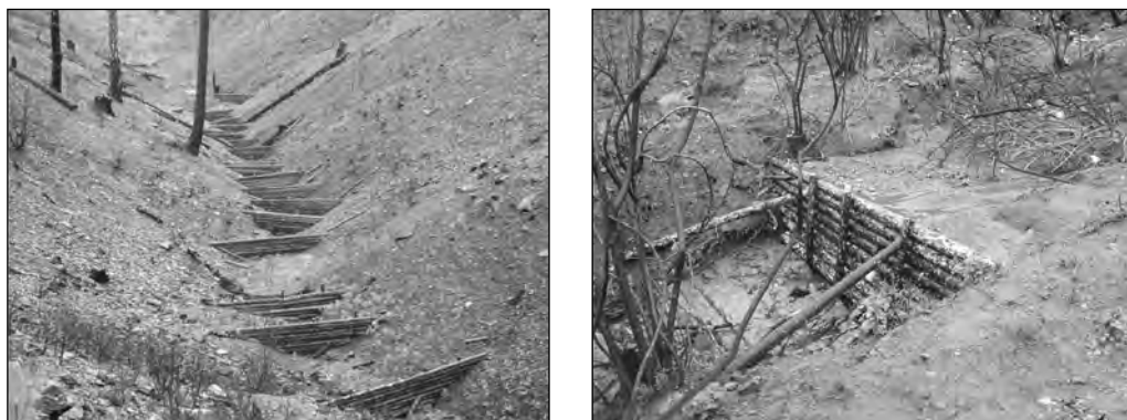
Figures 3a and b. A series of wood barriers (a) and withholding of sediments (b) in the forest of Taygetos.
